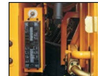
Centralised Electric Box for Single Point Trouble Shooting
